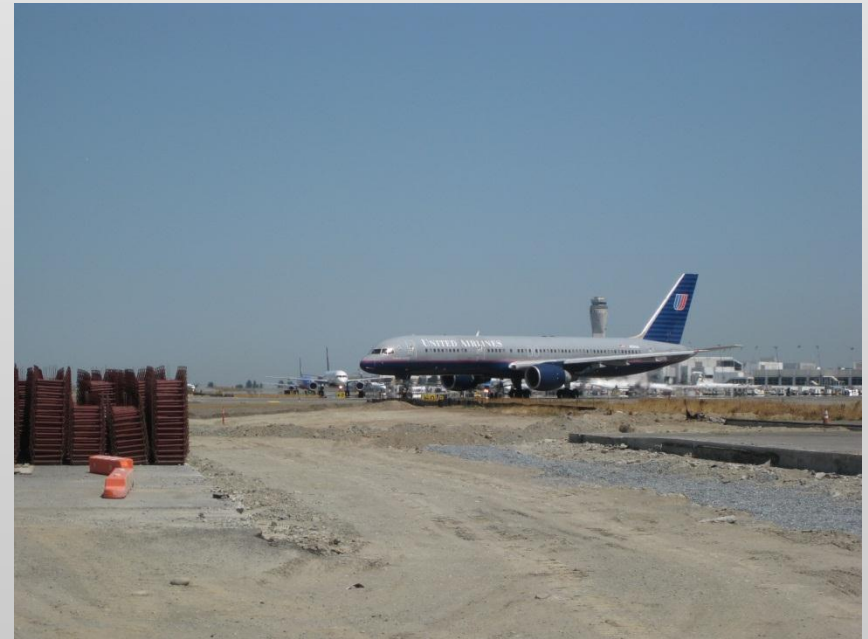
Runway 16C/34C Reconstruction
